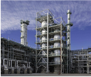
Fig. 1. Environment for service climbing robots. Sines refinery in Portugal.
